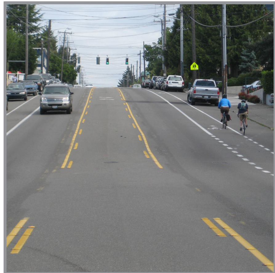
Lane Diet (Narrowing Travel Lanes to Accommodate Bike Lanes)
