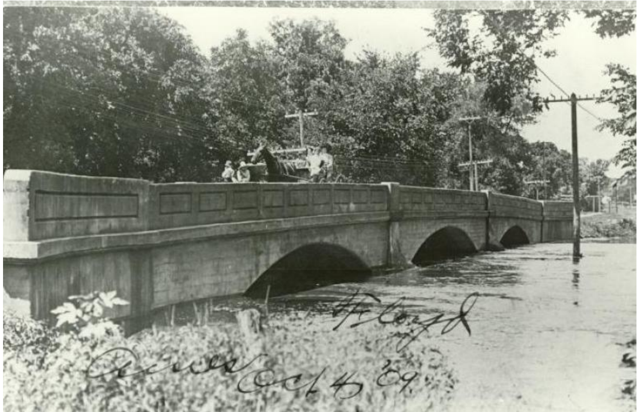
Historic Image 42: Lincoln Highway bridge over Ioway Creek. Within the year of construction, this flood water threatened the stability of the bridge, 1909.
