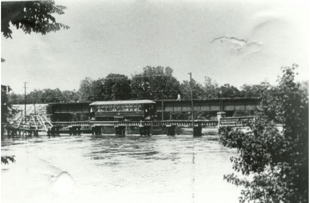
Historic Image 41: Remnant pieces of the foot bridge next to the streetcar on the left side, after it was washed away in the flood waters. 1918.
