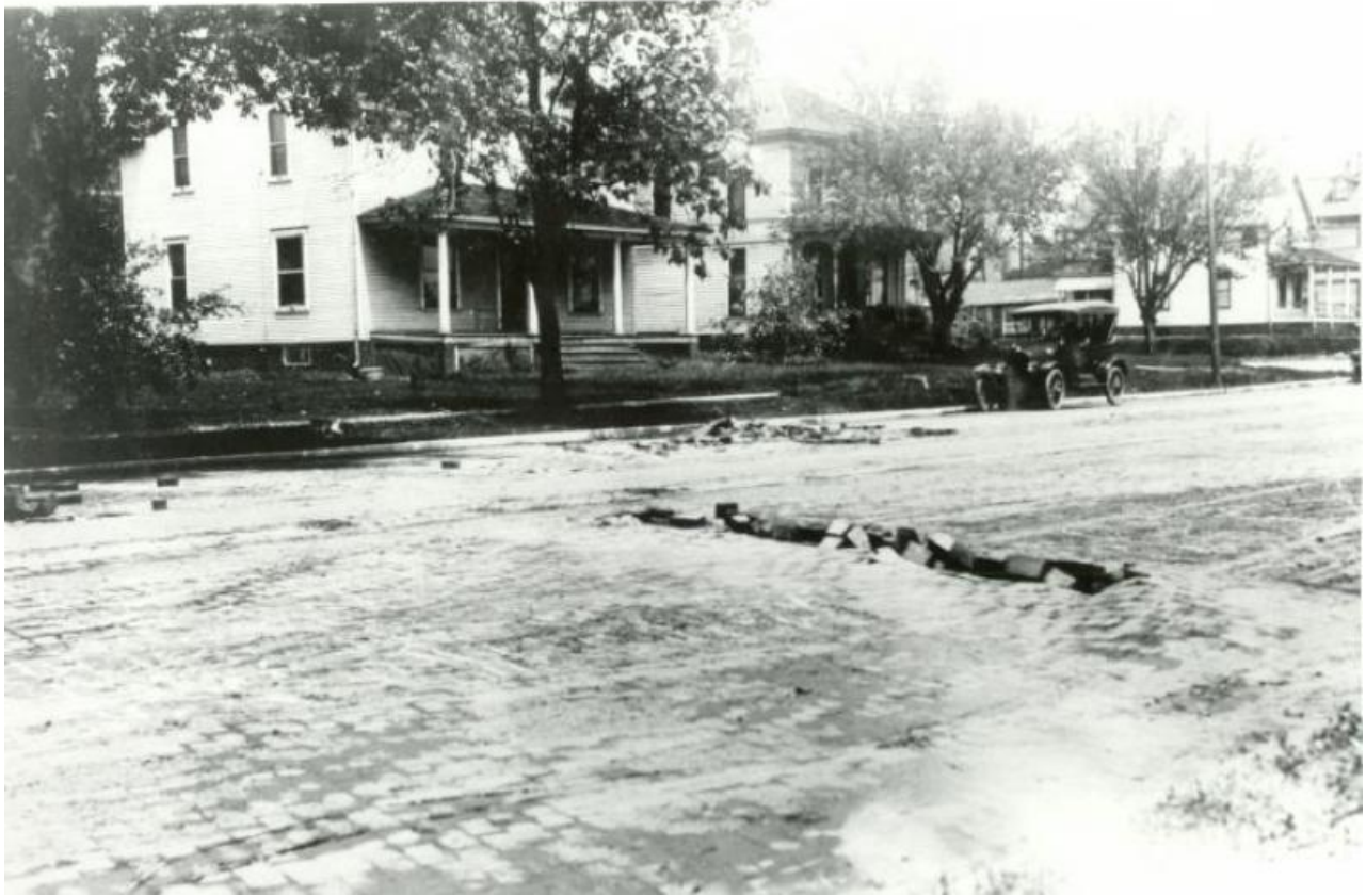
Historic Image 44: Wood “bricks” buckling as a result of freeze-thaw, water damage, and other weathering, 1918.
