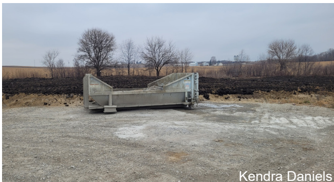
Rolloff washout container placed in flat area covered with gravel and accessible to concrete trucks.
