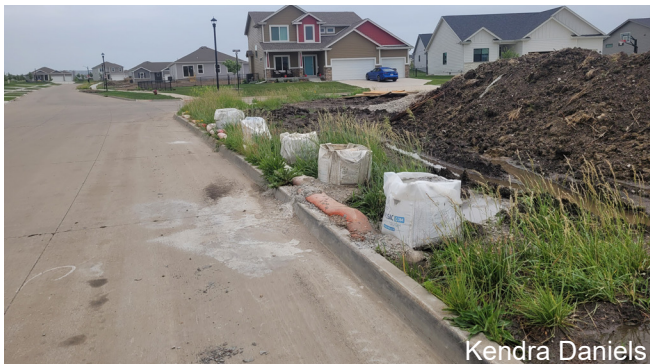
Multiple washout bags for ease of access. However, maintenance is required, bags are full, some overflow has occurred onto the street.
