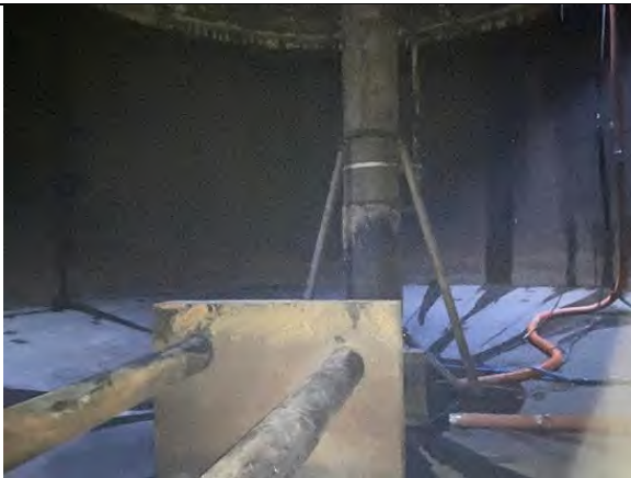
Interior of a primary digester during cleaning to improve performance and increase capacity.
