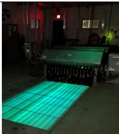
Ultraviolet (UV) Disinfection System
