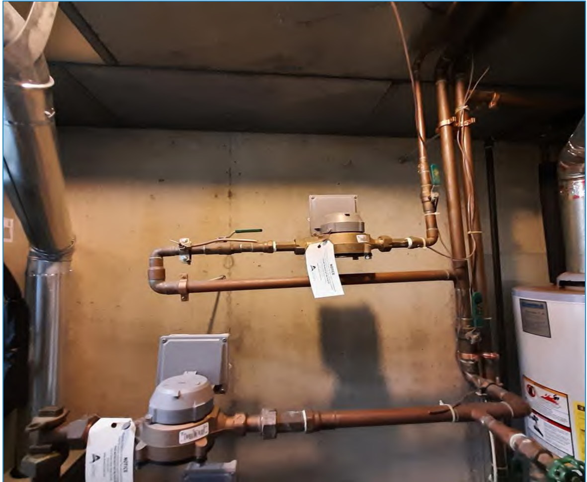
This photo shows a typical house and yard meter installation in an Ames home. The water flows through the house (lower meter) first, then any water that is used for outside purposes flows through the yard (upper meter).
