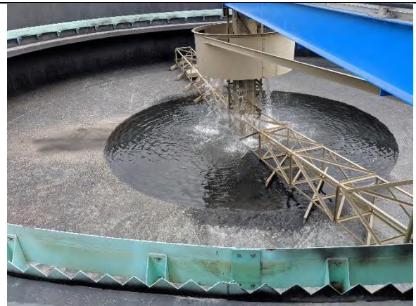
Clarifier being refilled after inspection
