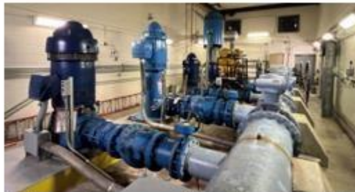
High service pumps at the old pump station
