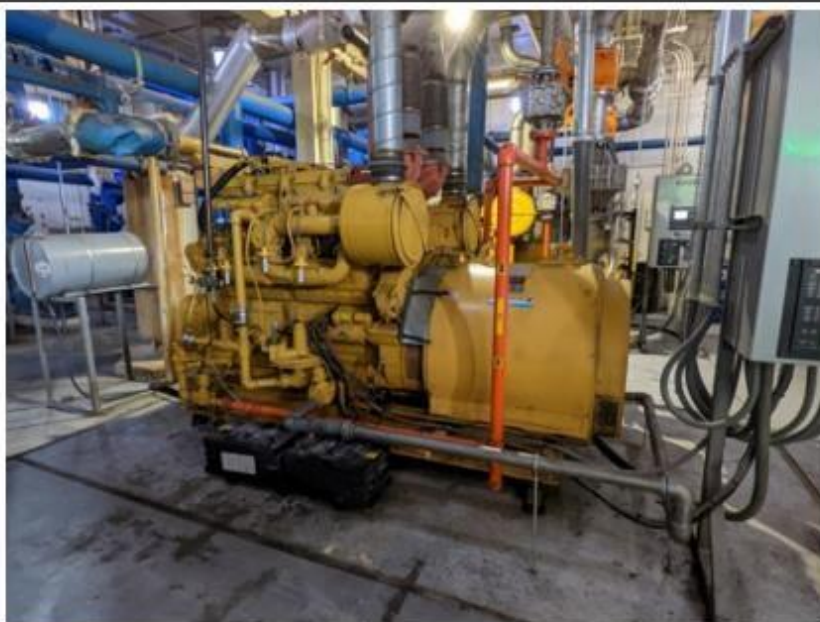
A methane engine/electrical generator unit at WPC
