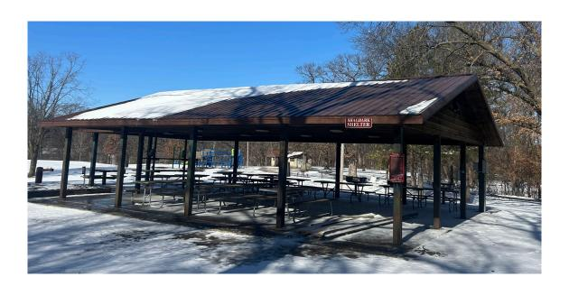
3. Heartland Roofing, Siding, and Solar, Des Moines, Iowa, completed the North River Valley Concession Stand Roof Replacement Project. The work included the removal of the asphalt shingles, underlayment, fascia, soffit, and replaced with all new underlayment, metal roofing, fascia, and soffit. See the picture below of the work that was completed.
